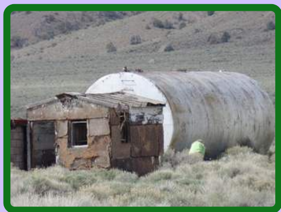
Photo of Above Ground Storage Tank in Round Mountain, Nevada for the former Carver's Station which received a site visit as part of a Phase I and II ESA.
